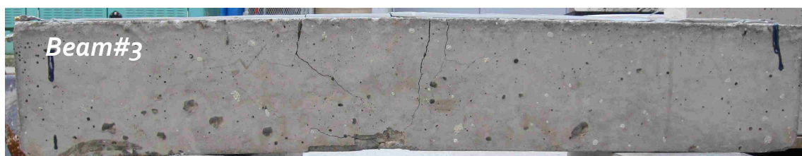
Figure A.2. Beam # 3_ Sika Grout 212_ Hold Tight ® 102
