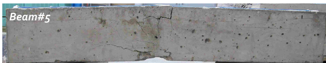
Figure A.4. Beam#5_ PC (mortar) _ Structural Epoxy
