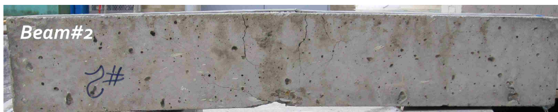
Figure A.1. Beam # 2_ PC -primer pretreated _ Hold Tight ® 102
